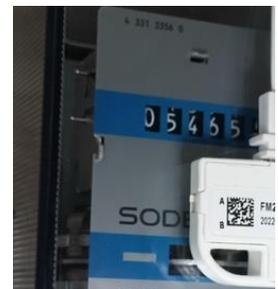
**Connect the white cable** to the FM442 battery/radio box (right side = orange panel).
